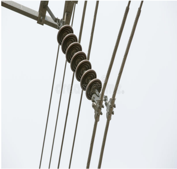
Fig 1.3 (b): Connection of Suspension type insulators
