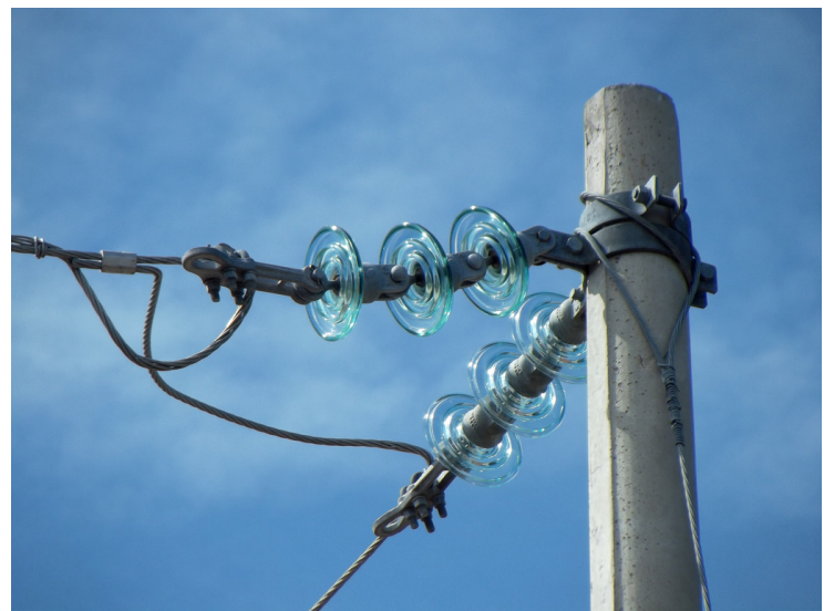
Fig 1.4: Showing the Strain insulators
