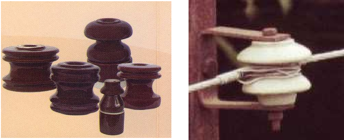
Fig 1.2: showing the spool/shackle insulators and its connection.
