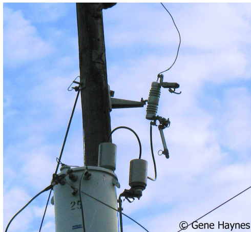
Fig 1.8: showing the drop out fuse
