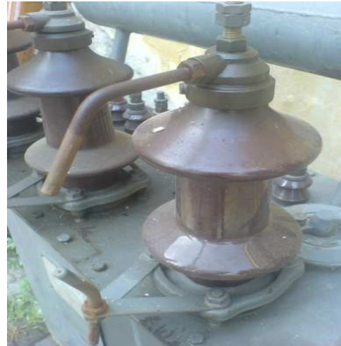
Fig.: Horn gap or Arcing horn
