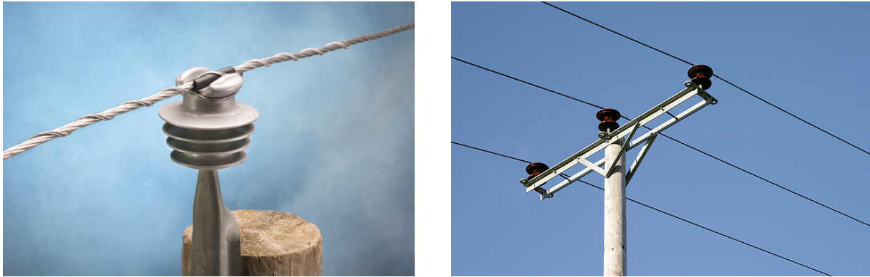
Fig1.1(b): Connection of pin type insulator.
